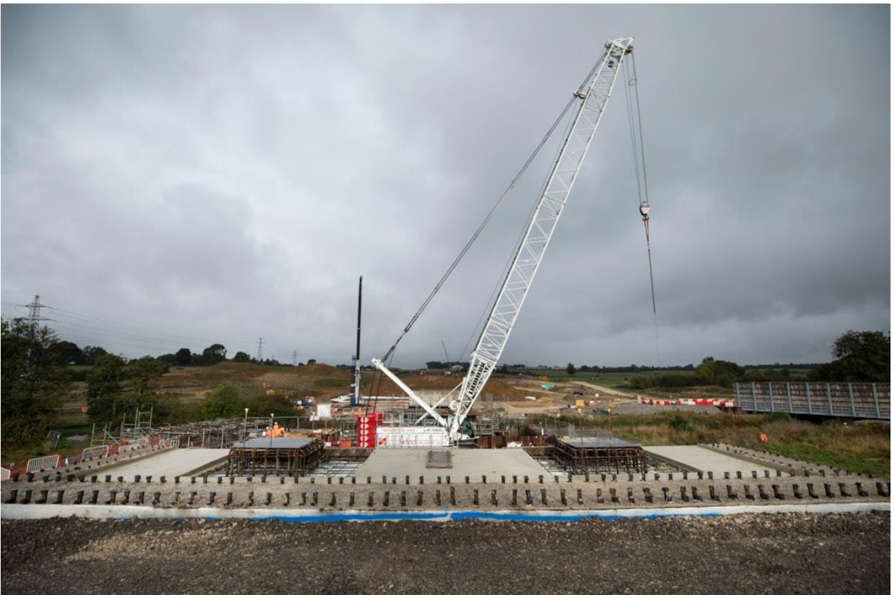
Figure 4: View from one of the completed abutments for the Turweston viaduct, October 2024.
