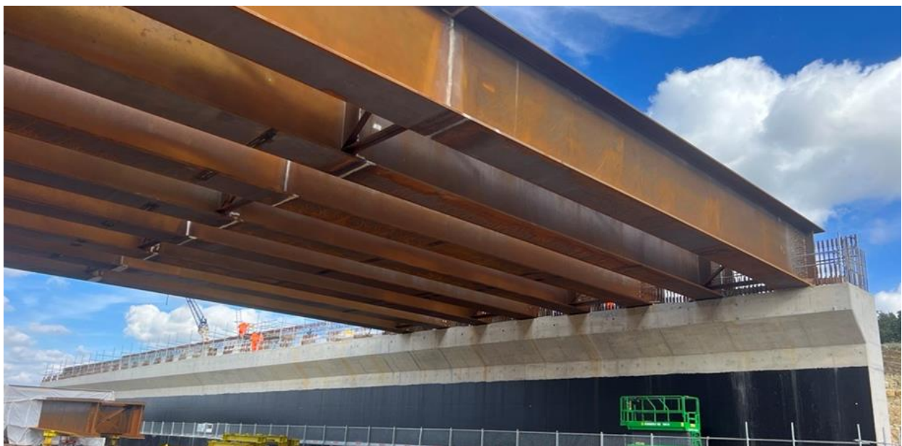
Figure 2: The image above shows progress on the installation of steel beams for the Turweston green overbridge, October 2024.
