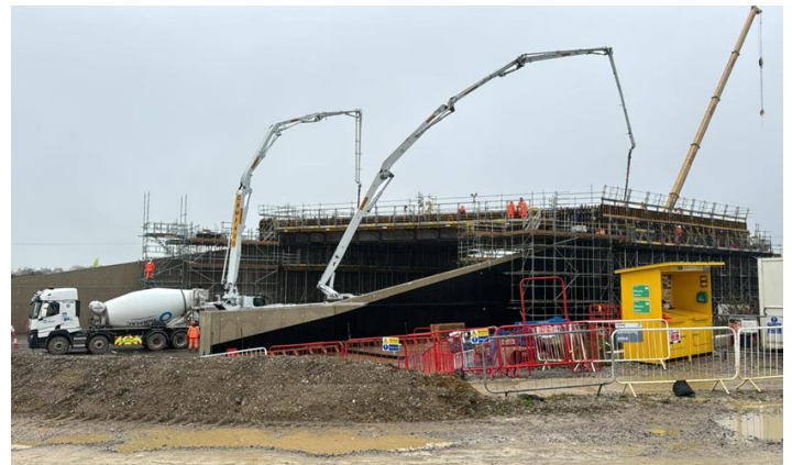
Figure 1: Teams at the Radstone Road overbridge conducted the concrete pour for the overbridge's deck in September 2024.
