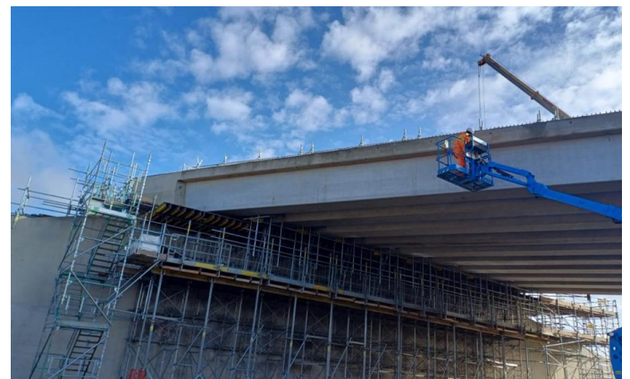
Figure 2: Radstone Road overbridge being prepared for the installation of the parapets, October 2024.
