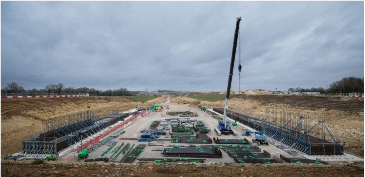
Figure 2: Construction of the Turweston green overbridge, September 2024.
