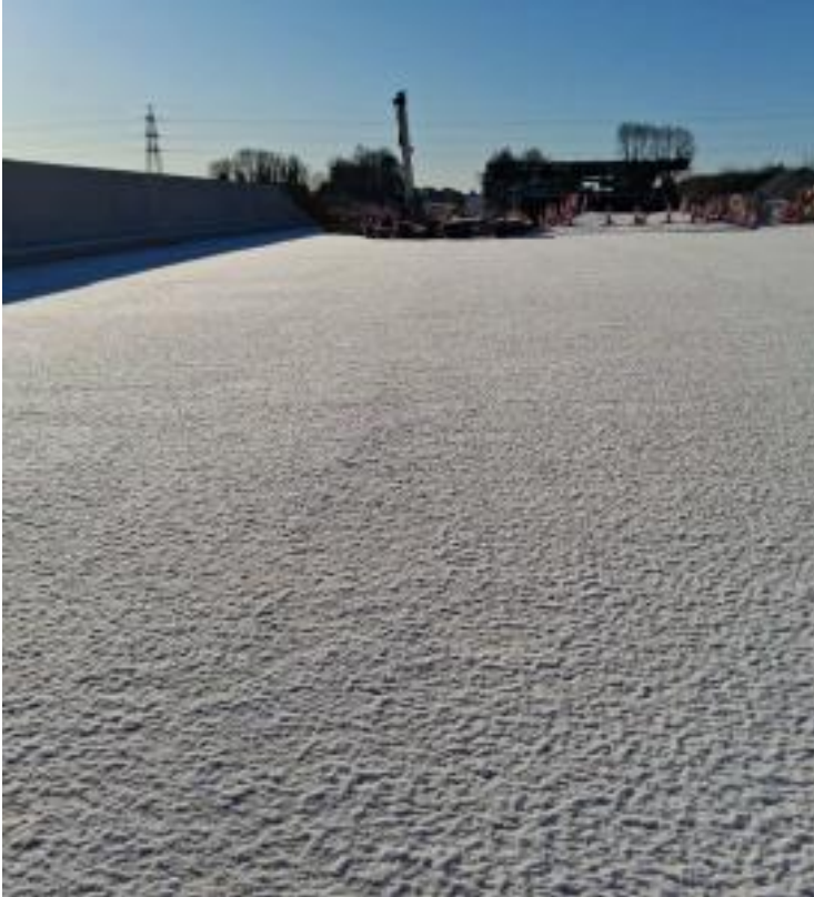
Concrete deck complete (Snow covering)
