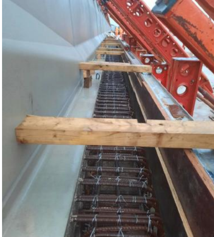
Parapet stitching continues
